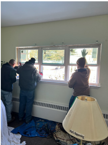
Workers from Nicholas Sears Construction install one of the new windows.
